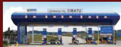
Direct Tol Gate KM 34.7
