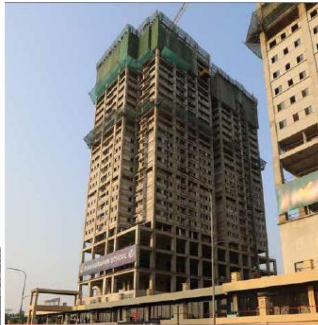
BLOCK 53022 Completed to Floor 29
