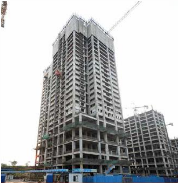
BLOCK 50021 Completed to Floor 28
