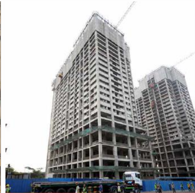
BLOCK 39021 Completed to Floor 24
