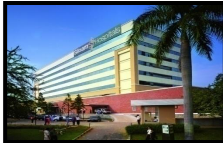
INT'L STANDARD HOSPITAL Siloam Hospital
